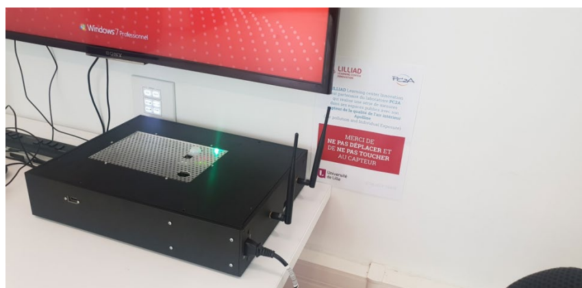
Figure 4. Sensor box in a workspace of the Lilliad Learning Center.
