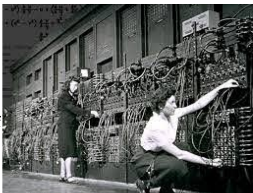
Fig. ?? . A view on the ENIAC with Marlyn Wescoff and Ruth Lichterman wiring the machine.
