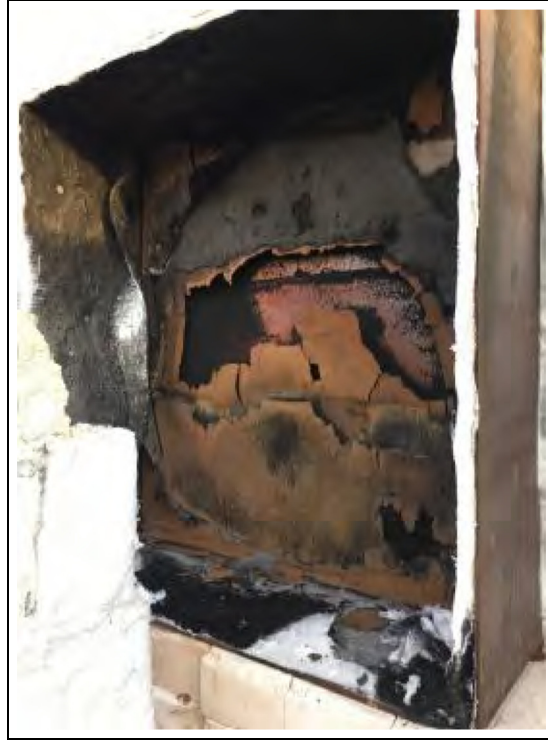
Figure 16. Picture after the large-scale jet fire test performed at Efectis, France.
