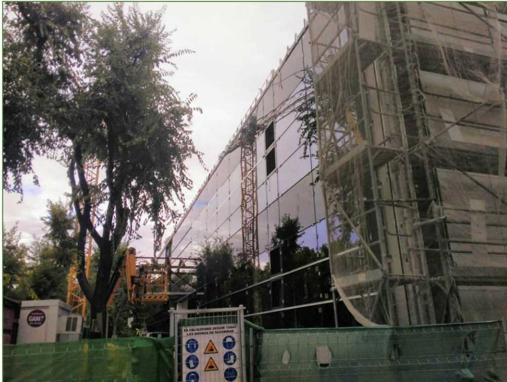
Figure 2 Current state of buiding works of the library, as of 20-09-2019
